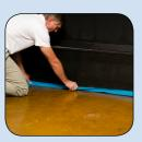
5 to 10 minutes. Any areas that dry prematurely should be sprayed again. Allow treated surfaces to dry before any additional procedures are initiated. After drying, remove any powdered residue using a stiff brush before continuing. At this point the floor can be polished and/or sealed. Polishing time will be reduced and less surface will absorb less sealer. Adjust procedures and/or applications appropriately.
